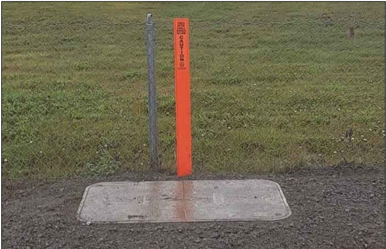
Picture 2: Typical Vault Buried Flush Following Construction
