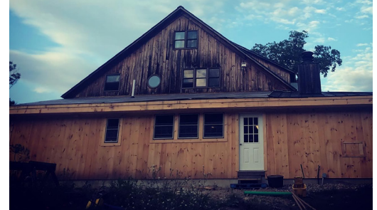
Above: The Orchard Hill Breadworks staff applies an ethos of teamwork to their craft and community relationships; Below: A 19th-century barn once owned by Noah Elbers’ grandparents houses the world-famous bakery & eatery.
