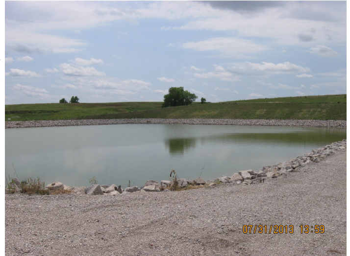
The new lagoon system in Ashton, NE.
