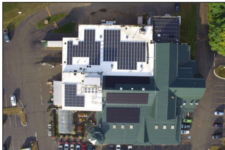
Aerial view of the solar array on Bishop's Orchards Market. Bishop's Orchard has a building array and ground mount solar array that provides 70 percent of the energy used.
