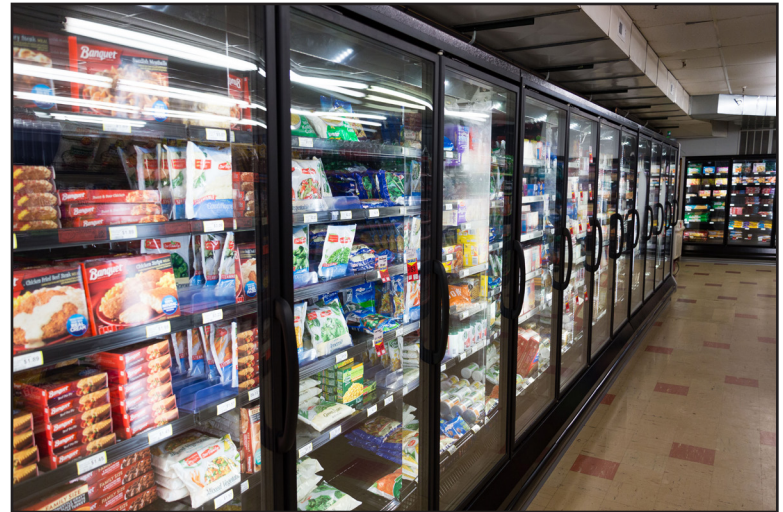
The new coolers in Oien Grocery improve energy efficiency and increase options for residents of the surrounding communities
