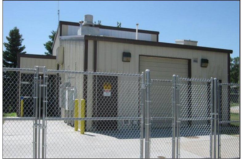
New Water Treatment Plant.
