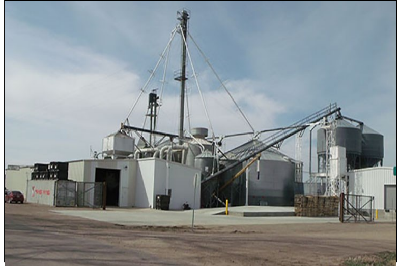
Clark Specialty Grains Processing Facility.
