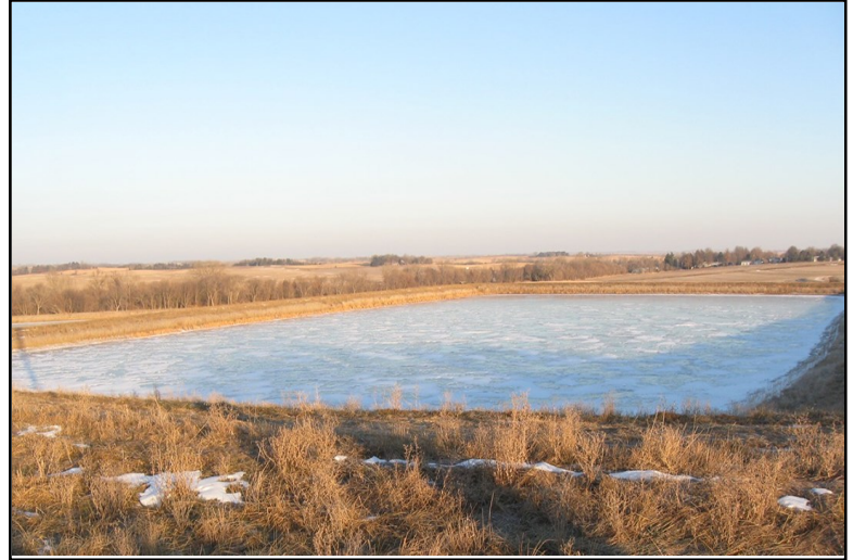
Davey’s new retention lagoon.
