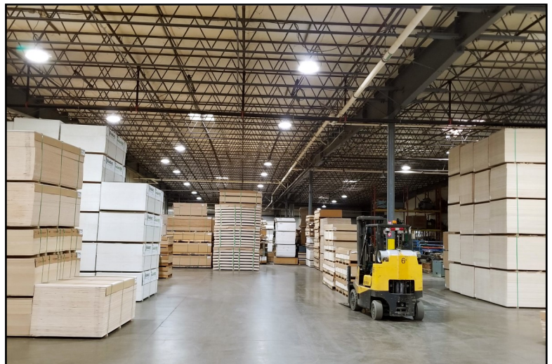
Precision Prefinishing installed energy-efficient lighting at its Harrisburg facility with help from a USDA grant.
