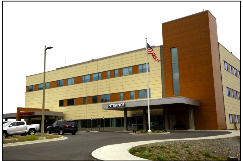
The state-of-the-art Curry General Hospital offers quality healthcare and expanded medical services in Gold Beach and the surrounding area.
