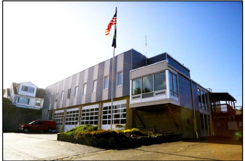
The fire station serving rural Depoe Bay on the Oregon coast received seismic improvements and was fully renovated with the help of USDA funding.
