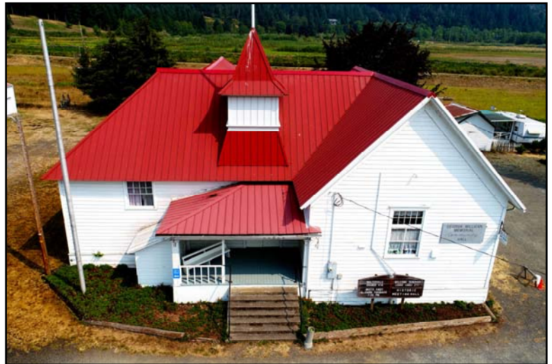
The roof on the Walterville Grange Hall was replaced with the help of a USDA grant.
