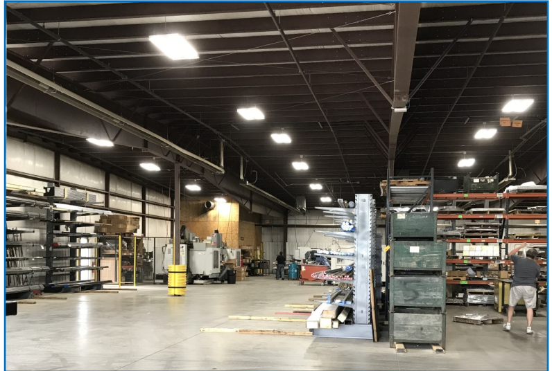
Pictured is the newly installed LED lighting inside the Dakotaland Manufacturing facility in Watertown, SD.
