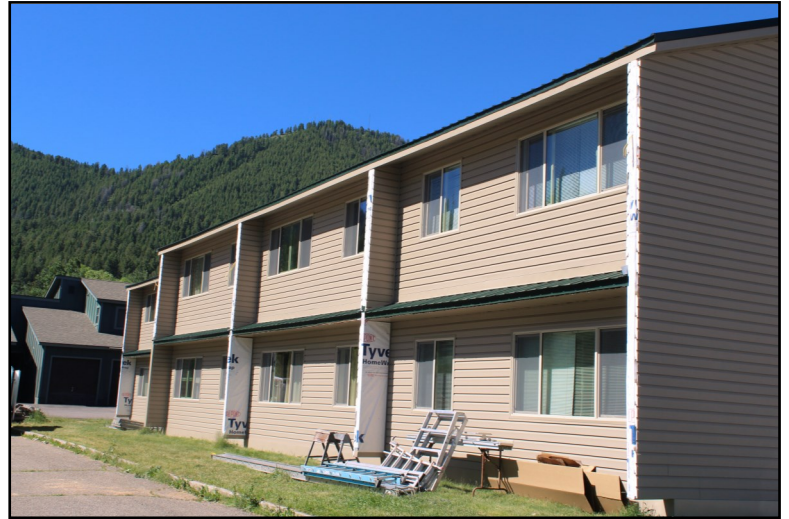
Renovation progress on Cedar Creek I Apartments in Jackson Hole, WY
