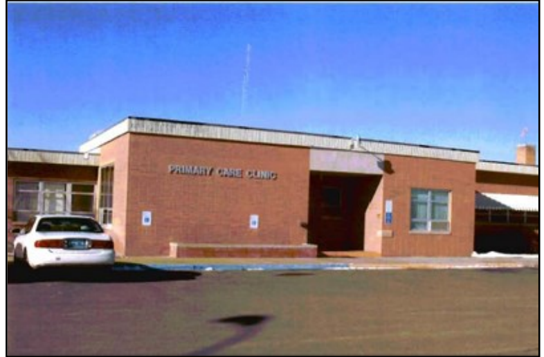
Front view of the current hospital built in 1956.
