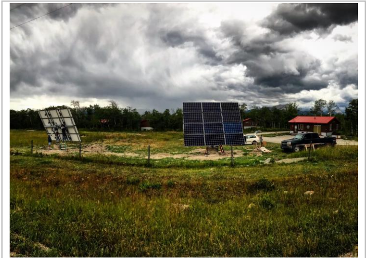
The 15,360 kilowatt-hours (per year) on-site solar array system generates about 90 percent of Park Cabin Company's annual energy needs. (Photo courtesy of Park Cabin Company)
