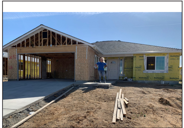
Sherry Parker poses for a photo by the construction of her new home in Northern California. Parker lost her home during the devastation of the Camp Fire in 2018. (USDA Courtesy Photo)
