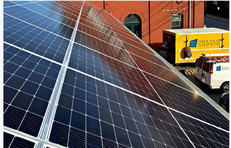
Biddeford-based Saco Bay Marine used an FY 2023, \$28,700 REAP grant to install a 19-kilowatt, roof-mounted solar voltaic system expected to meet most of the business's energy needs. The marine company is situated at Rumery's Boat Yard - built more than 60 years ago on the site of a coal-fired power plant dating back to the early 1900s.
