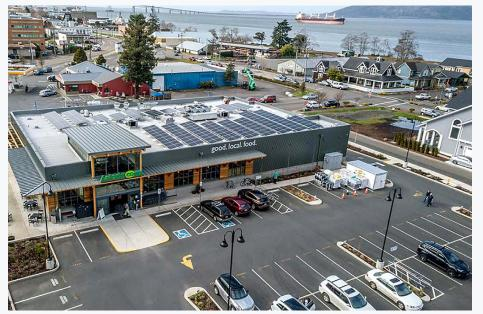
Astoria Cooperative is a local, community-owned grocery located northwest of Portland where the Columbia River meets the Pacific Ocean. Astoria used a nearly \$50,000 REAP grant to buy and install a 60-kW rooftop solar array – which generates energy from solar irradiance – even on cloudy days. The array is replacing roughly a quarter of the cooperative's monthly energy use. Success Story 4 Energy efficiencies help rural Kentucky grocery improve bottom line
