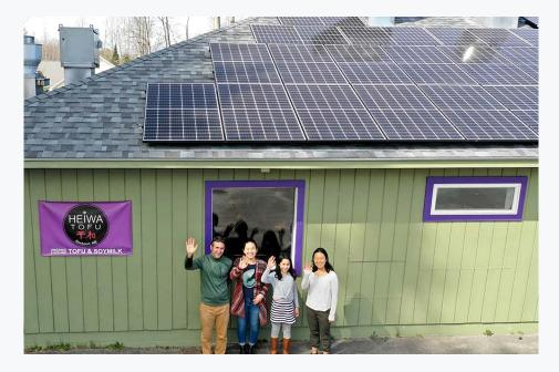
Camden-based Heiwa Tofu used an \$8,822 REAP grant to help them buy and install a 20.15 kW, roof-mounted solar photovoltaic system, which is saving them more than \$1,660 a year in energy usage.
