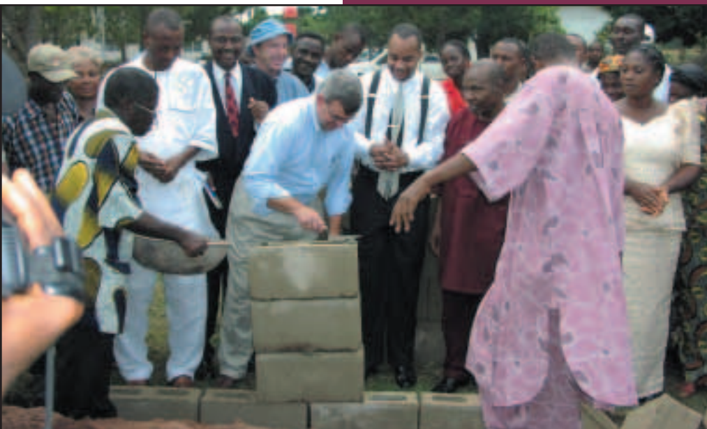
Jeff Jobe, co-op development specialist for USDA Rural Development in Iowa, takes a turn laying the foundation for the new Abia State Agricultural Business Development and Planning Center in Umhahia, Nigeria. USDA is supporting the center.
