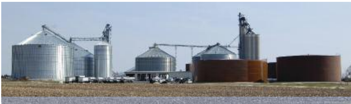
United Cooperative's South Beaver Dam (Wisconsin) facility is one of its largest grain locations. Two other Wisconsin co-ops recently voted to merge with United.
